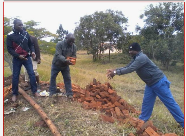
Student teachers and staff members passing bricks for construction
